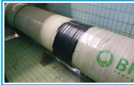
Floating pipe installation in water
